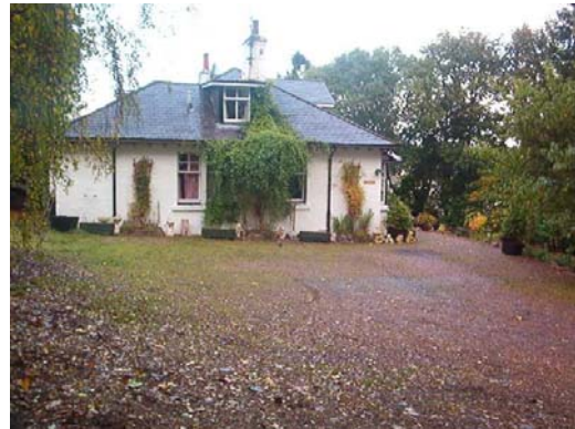
Fig 3 showing Kila (to be removed)
